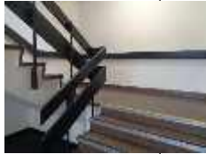
Good example of continuous handrails across a landing.
